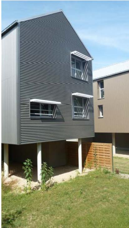
**Figure 1** : Example of two-storey house built on stilts. Saint-Pierre-des-Corps, France (CEPRI)
