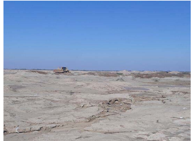
Fig. 8. Mechanical fixation by mud before rain season in September at SDS hotspot (Area 1).
