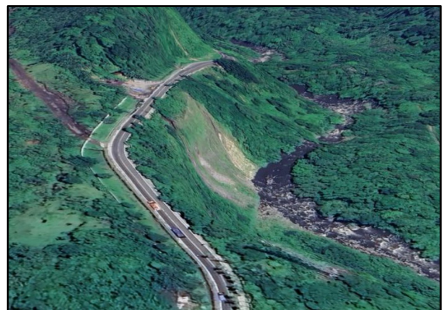
Fig. 1. Cliff condition before the landslide (source: google earth, february 23, 2024)
