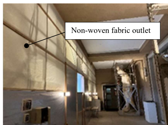
Figure 5. Interior view of the anterior room, including the non-woven fabric outlet for distributing dehumidified air.
