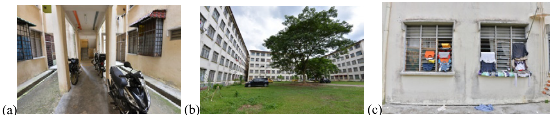
Figure 4: (a) internal corridor with parked motorcycles, (b) extended parking spaces on soft landscape and (c) clothes were hung on windows.
