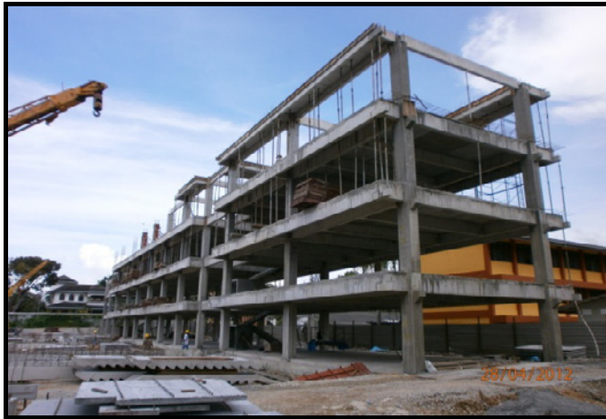
Figure 3: Erection of IBS Structure Component at Sekolah Kebangsaan Minden Heights
