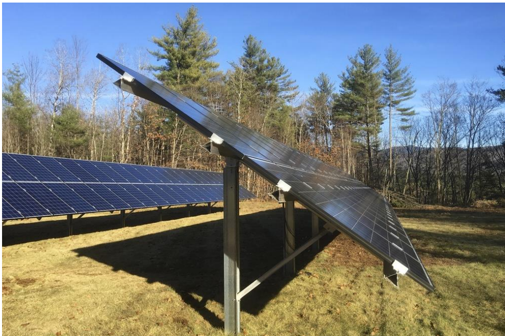
Fig. 1. Ground-mounted solar photovoltaic arrays at the Hubbard Brook Research Foundation. The system's estimated energy payback period of 2.4 years was significantly less than the simple payback period, 13.3 years. Note the driven-post system reaches soil depth of 2.4m, and requires no concrete to install.
