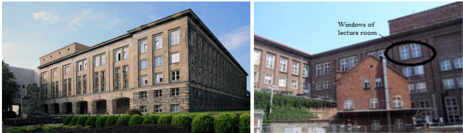
Fig. 1. View of inter-faculty laboratory-didactic building D-2 from front and from the internal courtyard side [15, 16].
