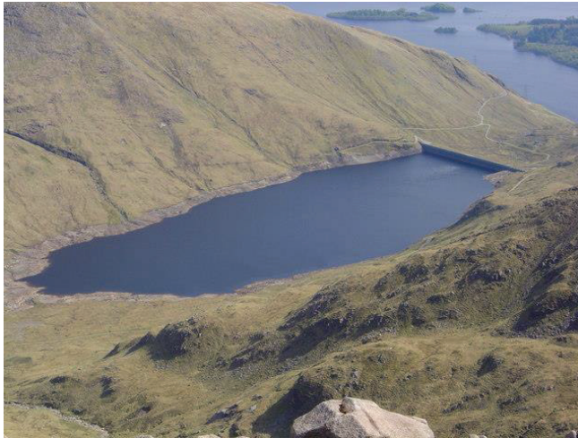
Figure 1. The upper lake and dam at Cruachan, above Loch Awe in Scotland, a 400 MW reversible-pumped water storage scheme commissioned in 1965.
