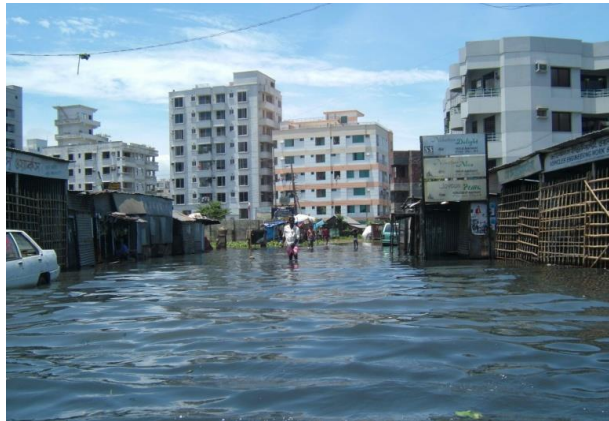
Fig. 9. 2004 flooding in the streets of Dhaka. (Source: CC BY-SA dougsyme).
