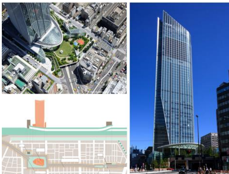
Fig. 2. «Toranomon Hills», Japan, Tokyo, 2014, 258 m, 52 floors, designed by Nihon Sekkei [12].
