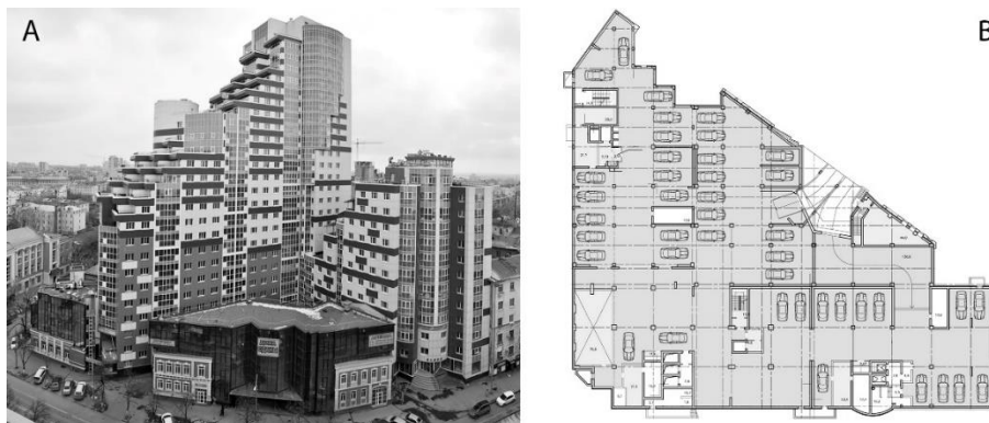
Fig. 3. Residential complex " Step Green House". A - overall view; B - plan of the underground floor (materials provided by the authors of the design).
