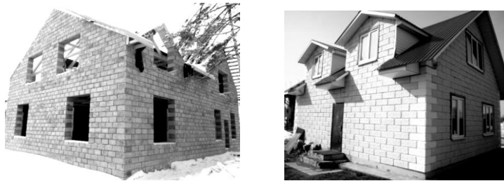
Fig. 3. Construction of the cottage with block
