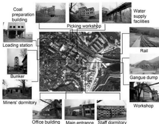
Fig.4-1 Current situation of industrial square facilities
