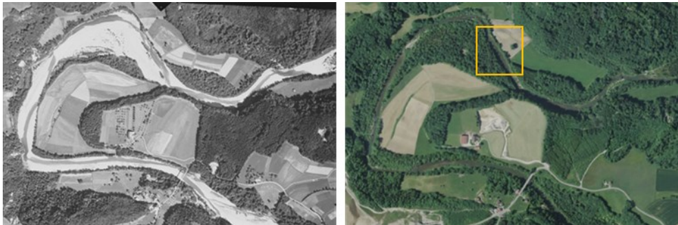
Fig. 1. Comparison of a meander at the Sarine residual flow section from 1943 (left) and 2012 (right). The active floodplain from 1943 almost disappeared. Nowadays, hardwood forest is present and the dynamic behavior of the river is strongly reduced. The yellow square corresponds to the location where the sediment replenishment was added (Fig. 2).
