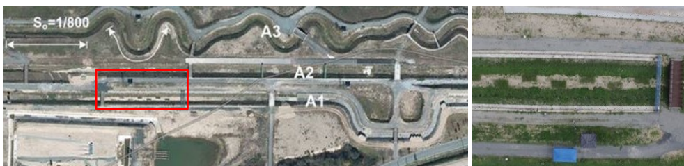
Fig. 1. KICT-REC Large-scale outdoor flumes (left photo) and red box indicates vegetation patches shown in the right photo (Flow direction ←).
