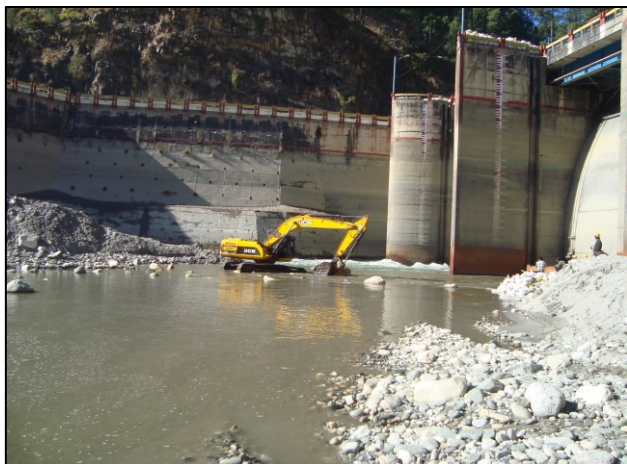
Fig 1. Sediment accumulation reduces storage volume and may interfere with the operation of dam outlet works. Removal of sediment by dredging or excavation (as shown in the photograph) may be needed to enable the dam to function.
