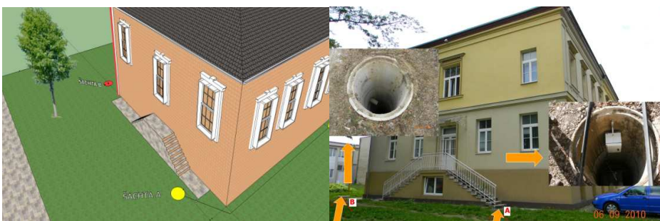
Fig. 5. Location of drainage wells near the PK6 building [5].
