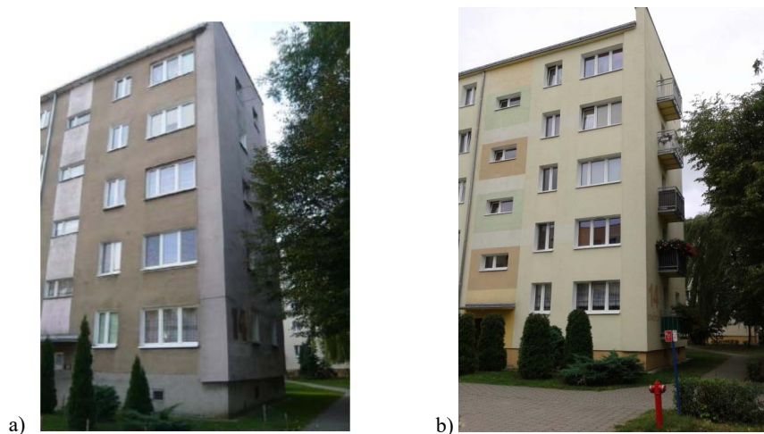
Fig. 1. Northern elevation of the building a) before thermo-modernisation b) after thermo-modernisation.
