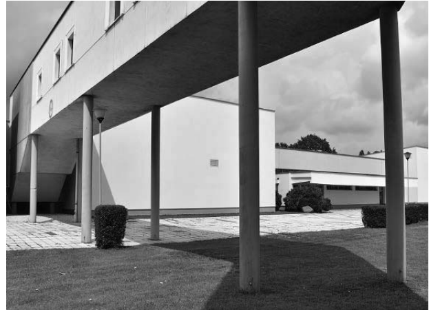
Photo. 2. The above-ground crossing between buildings.
