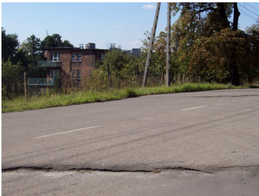
Fig. 1. Typical ground step created as the effect of mining of several coal seams to the border of protective pillar (photo by R. Ściagała).
