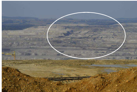
Fig. 1. Landslide in the open pit mine “Turów” – 2016 [3].
