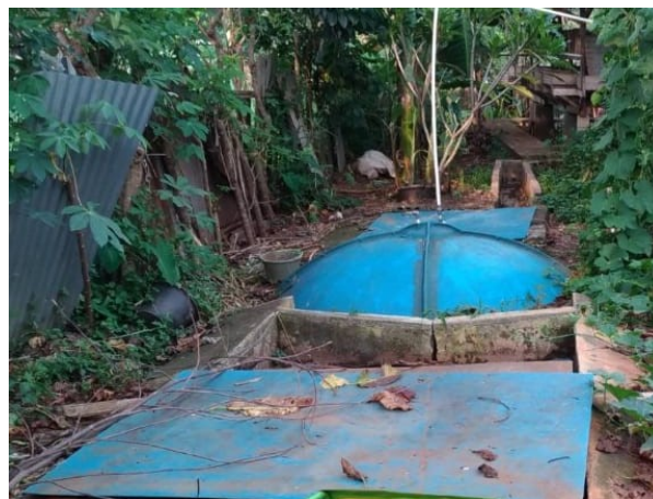
Fig. 2. Biodigester used in the present experiment at local farm in Depok, Indonesia
