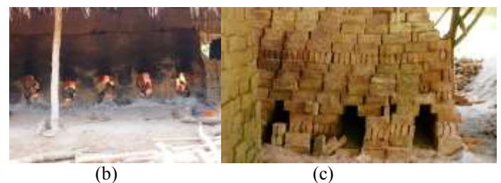
Fig. 3. Traditional batch kiln in Pedurungan Kidul constructed from the bricks
