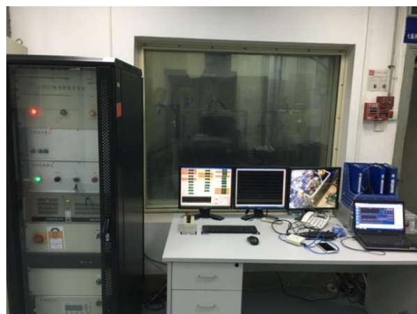
Fig. 4. Measurement and control system.
