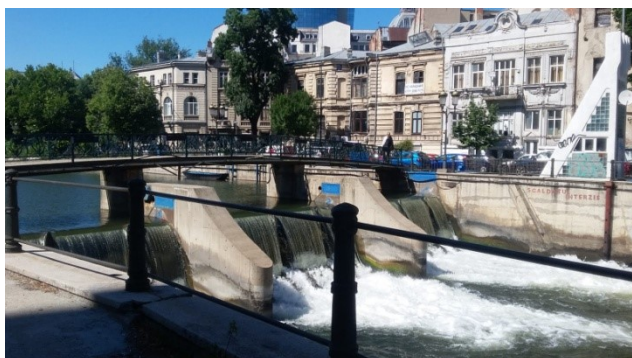
Fig. 4. Typical control structure with three gates (10. Operetă).
