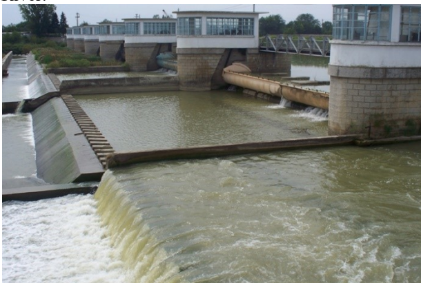
Fig. 1. Crivina- Ogrezeni dam and gates.
