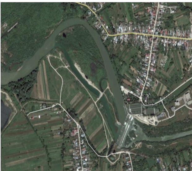
Fig. 3. Diversion dike and sediment deposits in Crivina-Ogrezeni reservoir.
