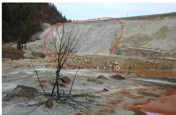
Fig. 5. Novat TDF – area of breach from March 2000
