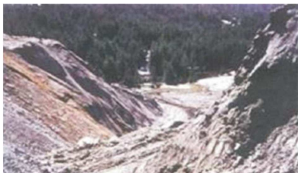
Fig. 4. Breach - upstream view
