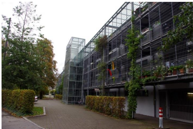
Fig. 2. The dwelling reconstruction with the false facade for vertical gardening - Konstanz, Germany [photo by author].
