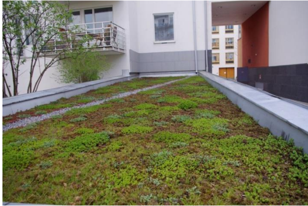
Fig. 1. Operated underground parking roof with easy care plants in the yard area of Hammar by Sjostad residential area in Stockholm, Sweden [photo by author].
