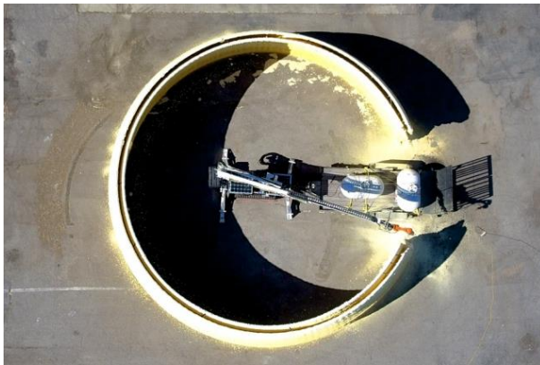
Fig. 2. The process of permanent printing formwork using 3D-printer MIT [4].
