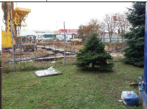
Fig. 5. Location of the sensor, making gravel columns.
