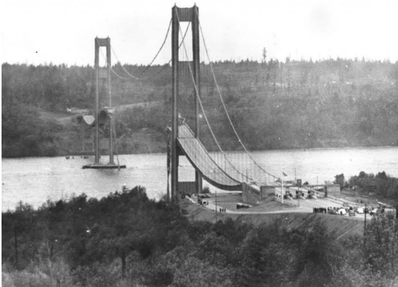
Fig. 1. Destruction of the Takom Bridge.
