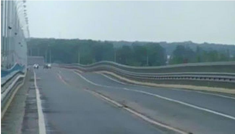
Fig. 2. Destruction of the Volgograd Bridge.
