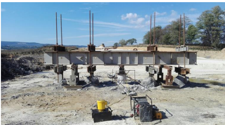
Fig. 1. Static Load Test (SLT) testing appliance anchored to adjacent piles
