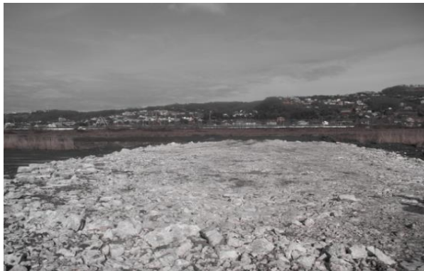
Fig. 3. Dumping of marl-and-limy soil on the pilot site H (the northern part of the quarter). The thickness of the layer of dumping is from 0.5 to 1.6 m
