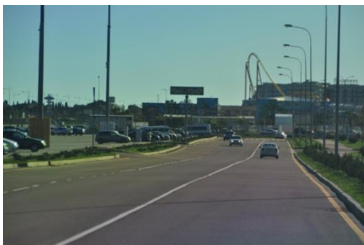
Fig. 5. The smooth sedimentation (to 0.9 m) of the roadbed as the result of residual consolidation of soils of the basis and carbonaceous soils of the embankment is visible essential
