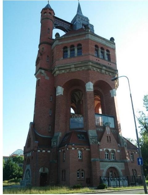
Fig. 1b. Water tower at al. Wiśniowa in Wrocław (Source: Biernat M., Stachyra A.K., 2017)
