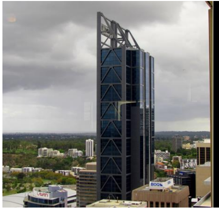
Fig. 4. High-rise Brookfield Place Tower in Western Australia
