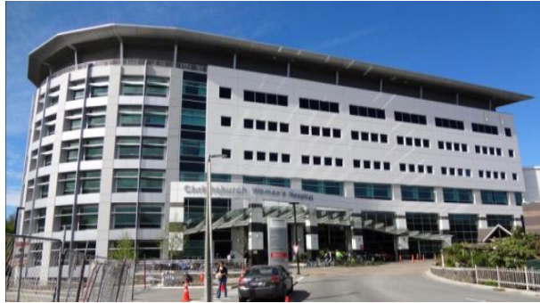
Fig. 6. Women's Hospital in Christchurch (New Zealand)
