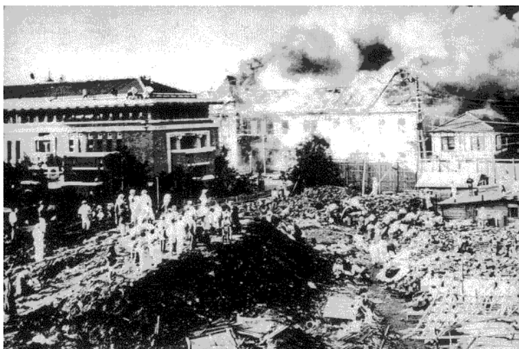
Fig. 2. Destroyed buildings near the hotel by the earthquake M_w 7.9 – 8.2 (September 1923)
