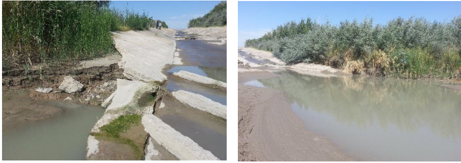
Fig. 3. Deformation processes at the interface of the inlet channel with the reservoir basin
