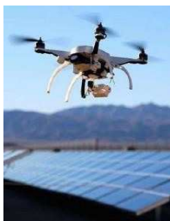
Fig. 1. Drone flying over a PV plant.
