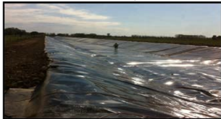
Fig. 2.2. – Geosynthetic membrane-lined irrigation canal.
