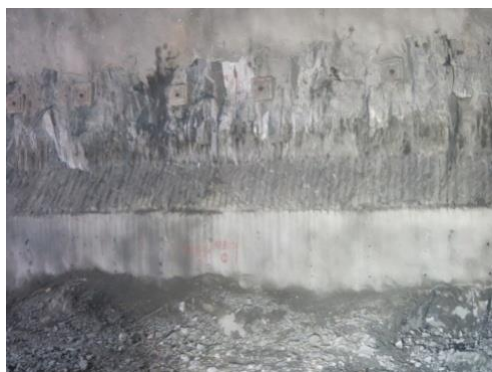
Fig.1. Excavation exposed face at rock-bolted crane girder
