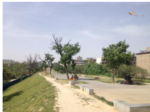
Fig. 3. The southern part of the eastern city wall and the southern part of the relic park are protected by covering with soil
