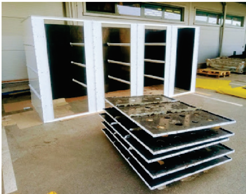
Fig. 7. Rubberizing of filters (source: WP systems s.r.o.).
