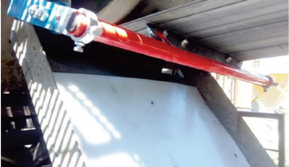
Fig. 5. Wiping technique (Source: WP systems s.r.o.).
