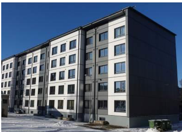
Fig 1. Overview of the reference building in 2015 before (above) and in winter 2017 after (below) the nZEB renovation.
