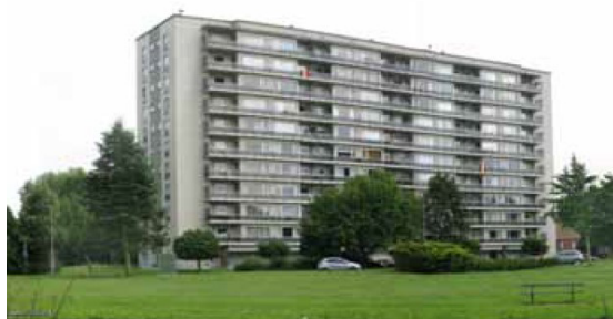
Fig. 1. Building IV before renovation.
