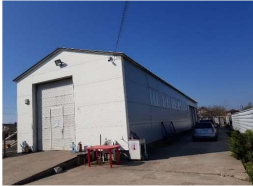
Fig.2 Industrial hall on which the experiment was carried out
