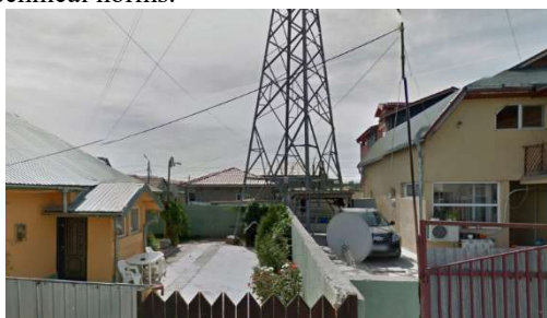
Fig. 1. OHL post with foundation within the premises of an inhabited building
