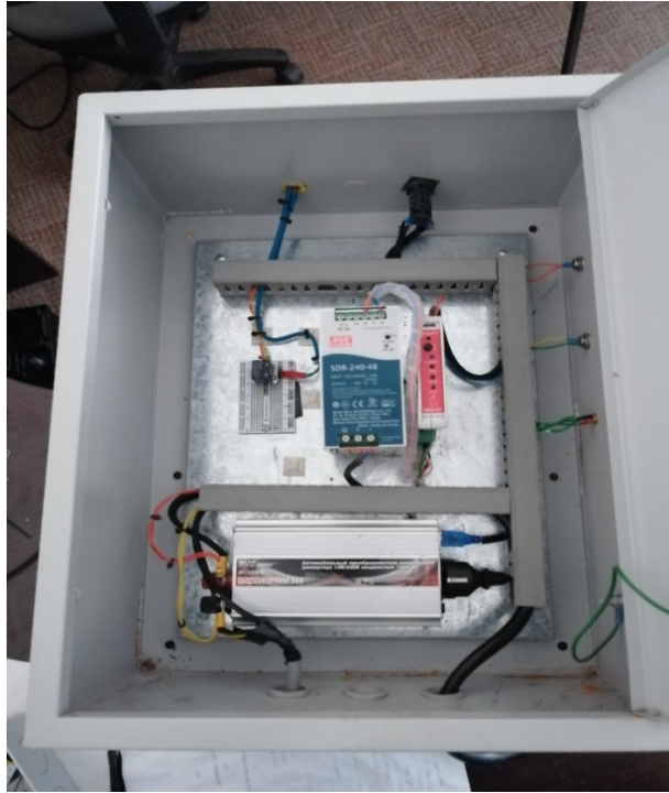
Fig. 7. Power section of an automated seeding system.
