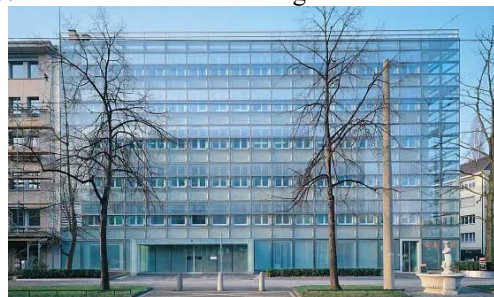
Fig.4. The SUVA office building after renovation
