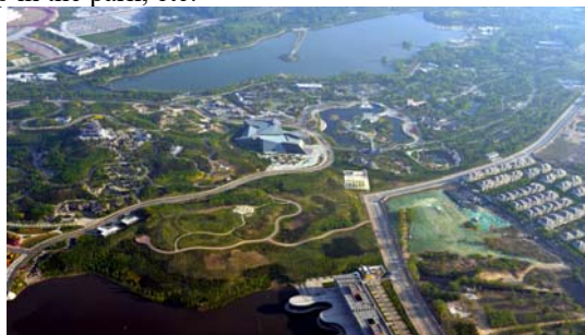
Fig. 2 urban wetland subsidence caused by coal mining in Nanhu, Tangshan
