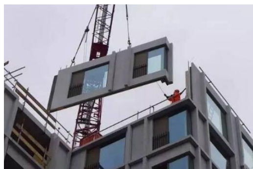
Fig.1. Construction site of prefabricated assembly components
